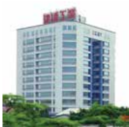
HEADQUARTERS Located in Taiwan
