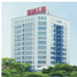
HEADQUARTERS Located in Taiwan
