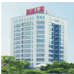
HEADQUARTERS Located in Taiwan
